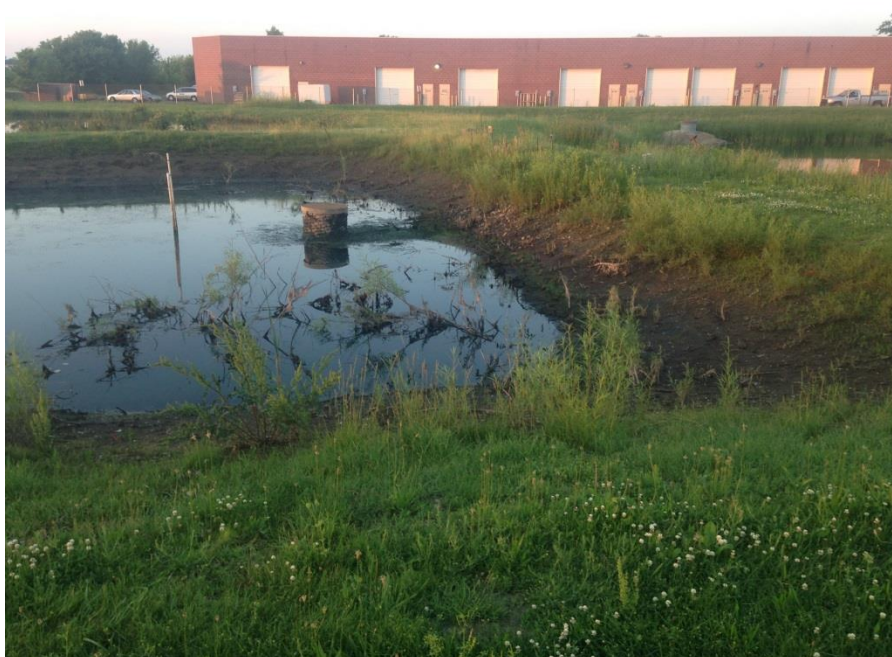
Figure 9. The same detention basin as shown in Figure 8 24 hours following a June 2014 rain event that filled the basin.
