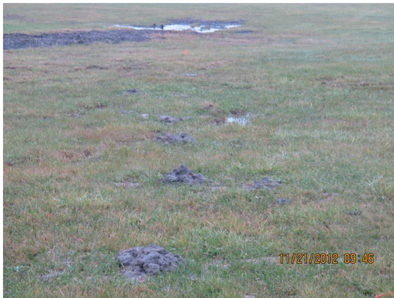
Figure 7. Mounds of soil after installation of EGRP ® units associated with detention ponds at Detroit's Mettetal Airport.
