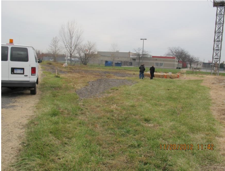
Figure 4. Problematic area holding water at DET.
